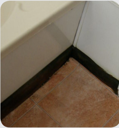
Regular cleaning will stop mould growth
